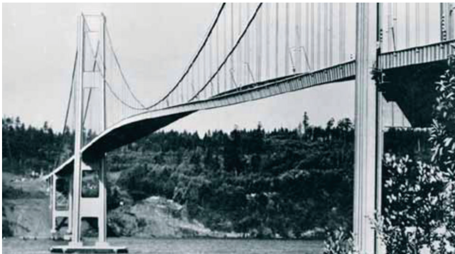
Fig. 7. The Tacoma Narrows Bridge in torsional oscillation on the morning of 7 November 1940. (from https://www.unirc.it/documentazione/materiale_didattico/599_2010_264_7525.pdf )
