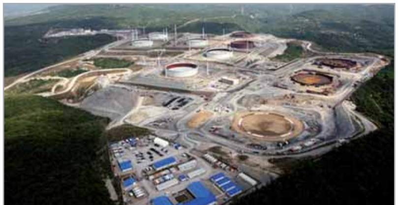
Fig. 1 - Tank farm at the CPC Marine Terminal
