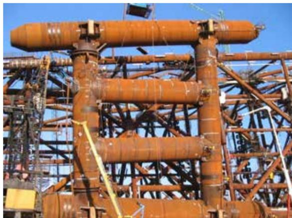
Figure 2 - Rolling-up of Large Auxiliary Buoyancy Tanks for Jacket free-floating
