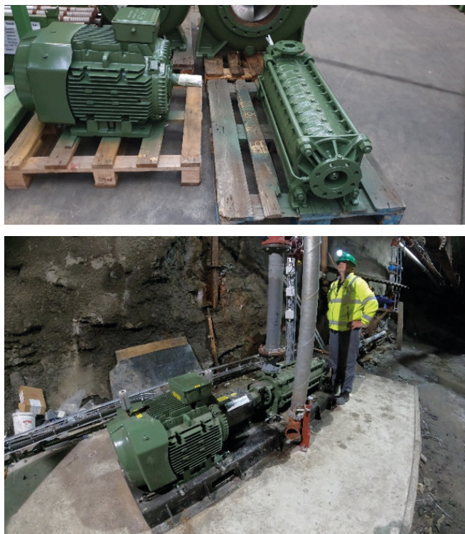
Fig. 2. SAER multistage turbine model E-TMZ-4P-50-80. Top: during manufacture; bottom: after installation.
