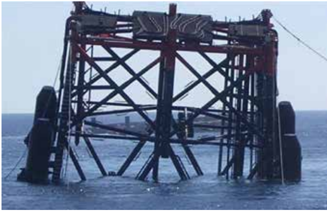
Fig.6. Sabratha jacket in free floating condition after the launch.
