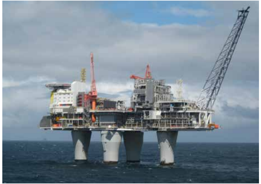
Fig. 1. The Condeep platform Troll A. (credit: https://commons.wikimedia.org/wiki/File:Troll_A_Platform.jpg )
