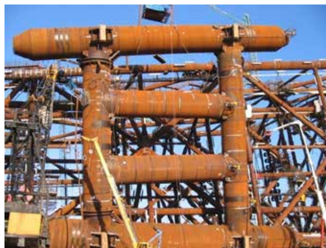
Fig.5. Sabratha jacket's auxiliary buoyancy tanks (ABT). The ABT design was created in 2010.
