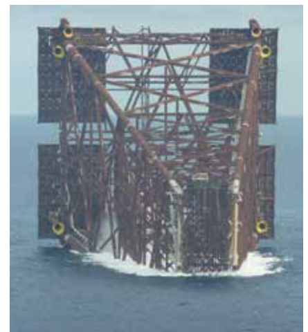
Tamar jacket launched from barge H851. (credit: https://commons.wikimedia.org/wiki/File:Tamar_jacket_launch_2.JPG )
