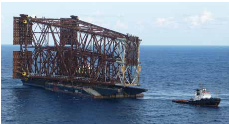
Tamar jacket on barge H851 with President Hubert on main bridle. (credit: https://commons.wikimedia.org/wiki/File:Tamar_jacket_on_H851.JPG )
