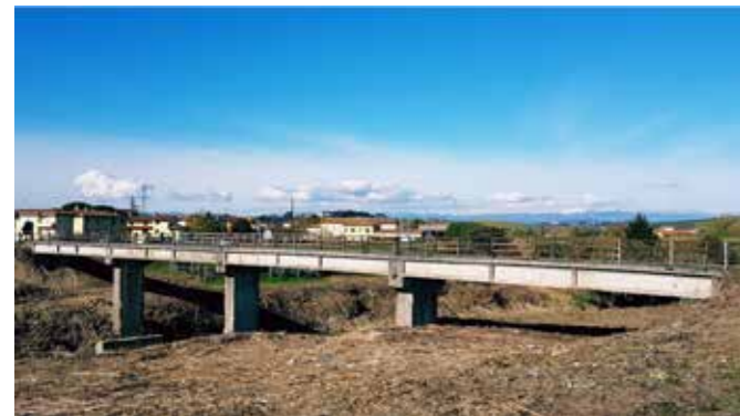
Figure 1 - The San Miniato bridge - Current conditions
