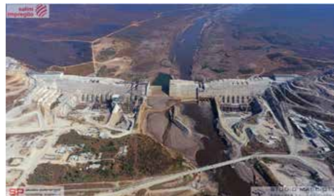
Fig.1 - GERDP Dam under construction
