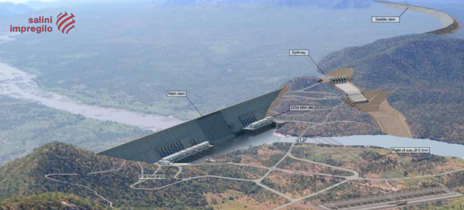
GERDP hydroelectric project, Main Dam general layout
