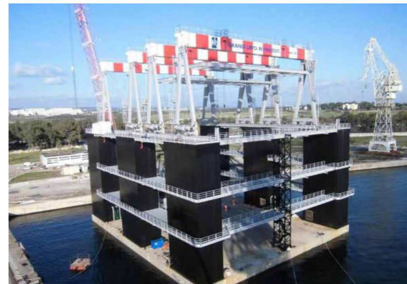
Fig. 1 - Gantry cranes on rails installed on a floating dock
