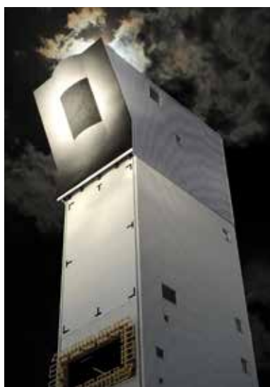
Solar Tower Julich (STJ)
